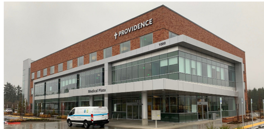
On demand, contract and 24/7 service for all brands of automatic doors
