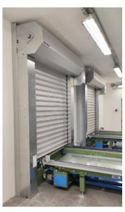
ASSA ABLOY RP2000 Rigid curtain opening speed up to 2.0 m/s, closing up to 1.2 m/s
